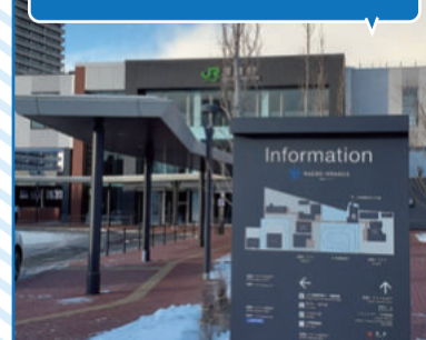
SP30 Naebo Station South Gate
